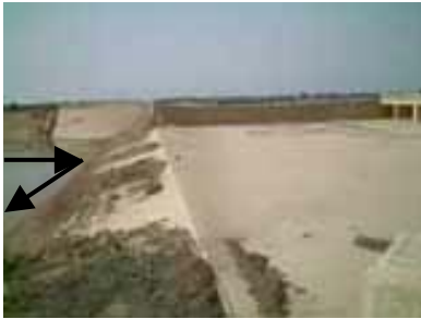
Above and below: entry to the super-passage is too high for floodwater to go over.
