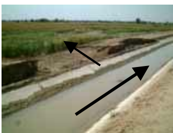
Top left: blockage to work the minor. Top right: distribution canal far below the level of farmland. Sump pumping is used for irrigation. Bottom: breaching from blockage.
