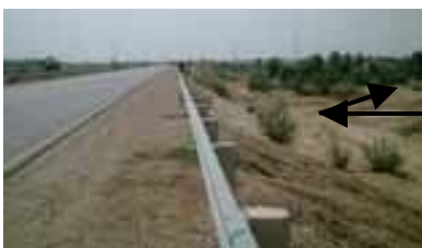
FCC disconnected by the Highway.
