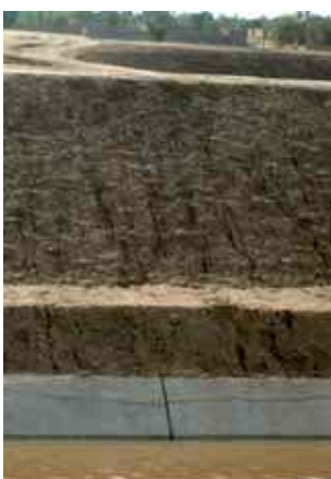
Cracks were present in almost all embankments
