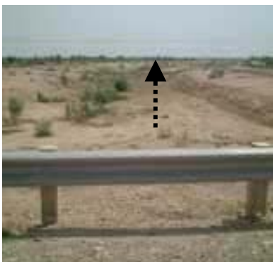
Disconnected FCC on the east side of the Highway. It is obvious that it has never contained water. Marks made by bulldozers are still present.
