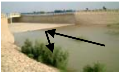
Above and below: entry to the super-passage is too high for floodwater to go over.
