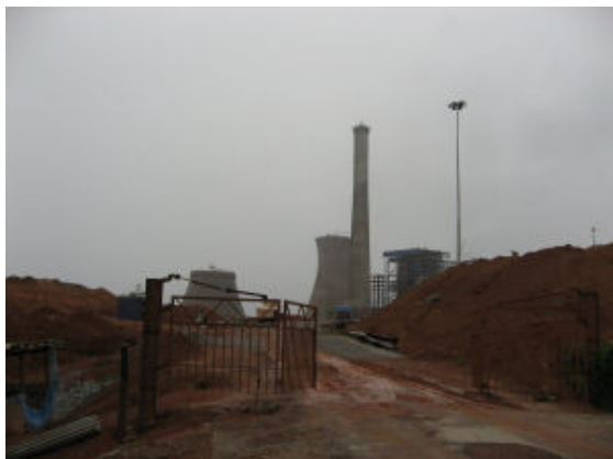
Photo1: Construction site of the power plant
