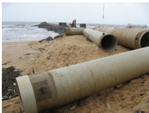
Photo 4: Construction site of the cooling water pipeline system
