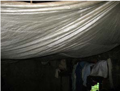
Photo: Sheet under the roof
