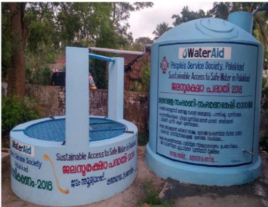
Photograph 2: Rain Roof water harvested into storage tanks and excess water is used to recharge open well
