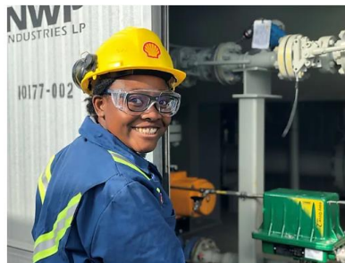
A worker inspects an electric actuator, introduced to reduce methane emissions, at Shell Canada's Groundbirch natural gas project.
